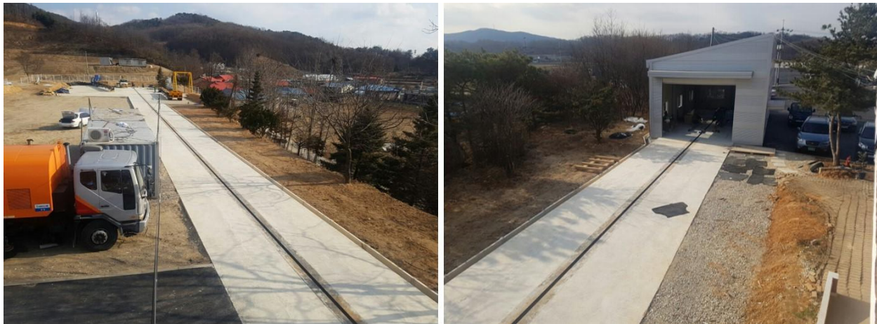
Figure2. Full scale crash test bed(Smart Air Chamber Co., Ltd.)
